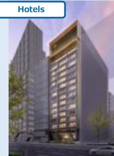
Ginza 7-chome Showa St. Development Project (2029)
