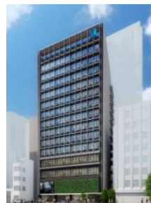
Hulic Toranomon No.2 Building
