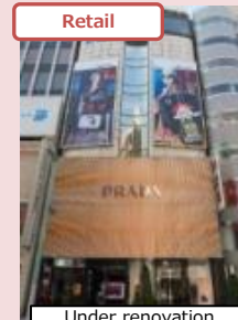
Under renovation World Town Building Renovation Project (2026)
