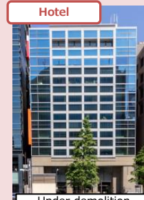
Under demolition Ginza 7-chome Showa St. Development Project (2028)
