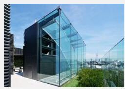
Hulic Head Office Building Rooftop Natural Ventilation System
