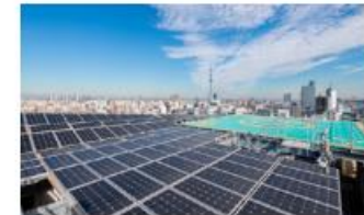
Hulic Asakusabahi Building
