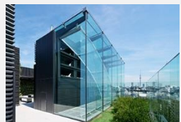
Hulic Head Office Building Rooftop Natural Ventilation System
