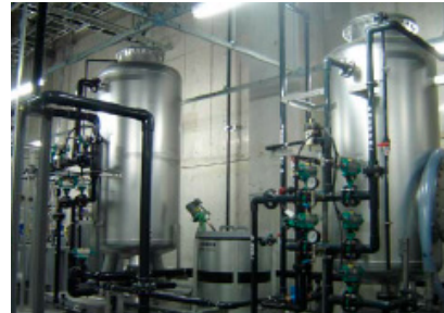
State of installation of subway seep water filtration system (Ochanomizu Sola City)
