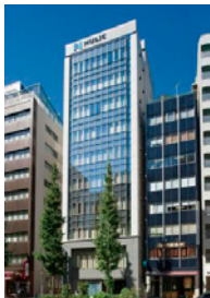
Hulic Kandabashi Building
