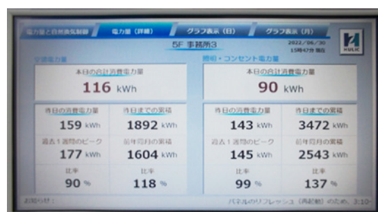
Energy management tool (Hulic Asakusabashi Building)
