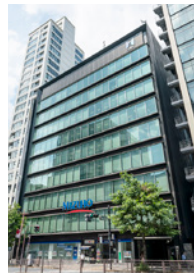
Hulic Kojimachi Building
