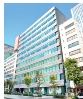
Hulic Toranomon Building
