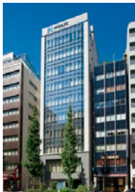
Hulic Kandabashi Building
