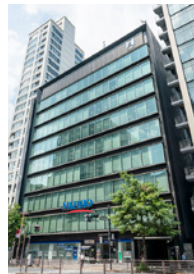
Hulic Kojimachi Building
